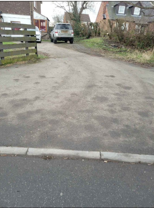
Site Photo Existing Dropped Curb
