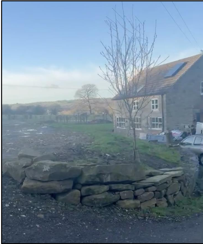
Figure 3: The C3 Building (Access looking W
