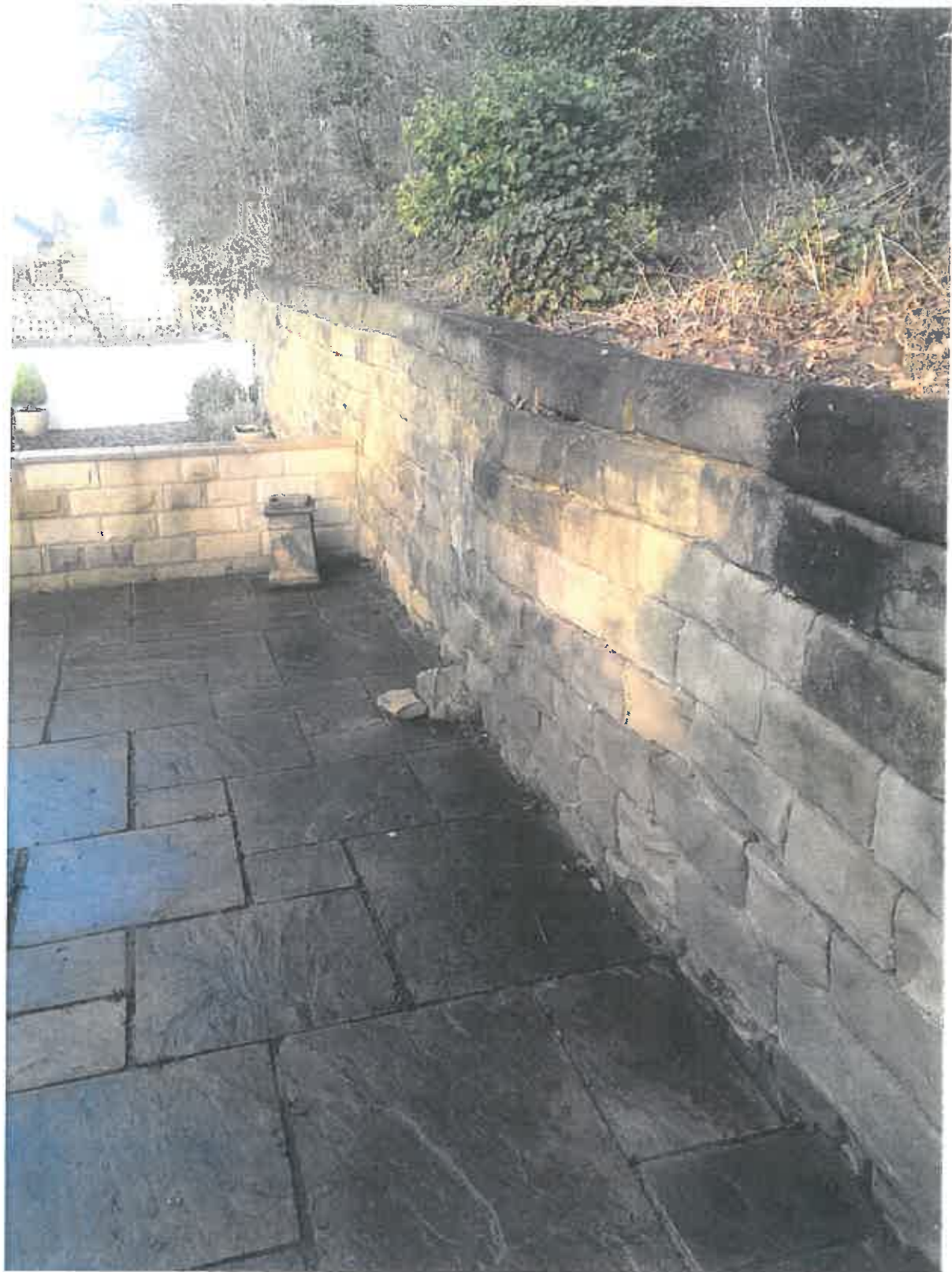
Photo 1 – Left Hand Side View towards No 85 from No 87 Showing Bulging and Misalignment to wall
