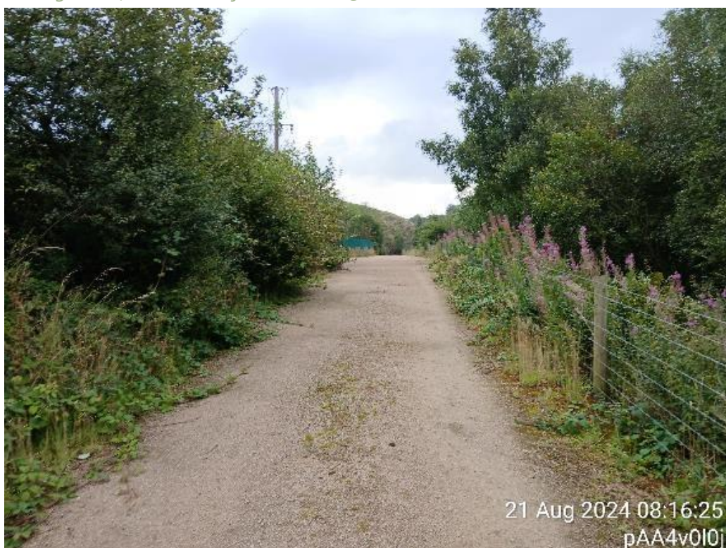
Plate 7. Artificial vegetated; unsealed surface area U1c-3
