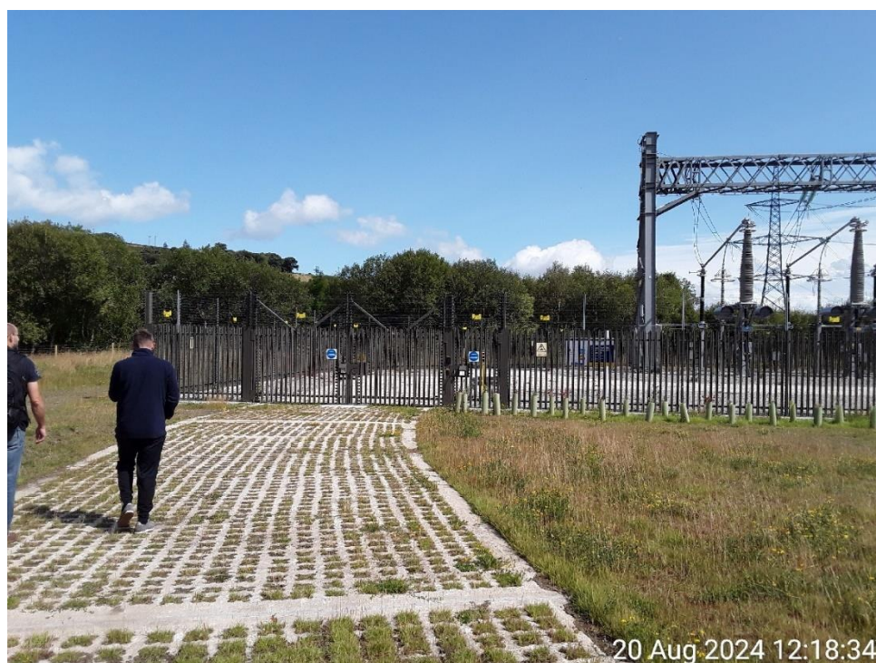
Plate 23. Sparsely vegetated land – ruderal ephemeral – New substation at Wogden Foot LWS
