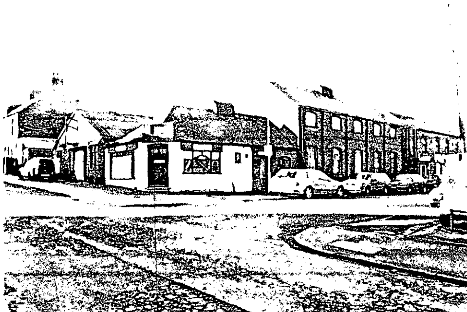
VIEW OF SITE FROM WELLBECK STREET
