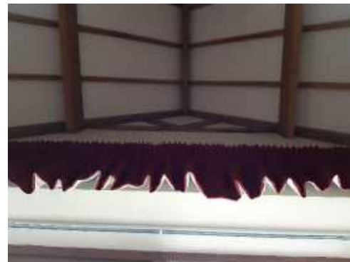
Photograph 10: B6 (internal view of gable end from below)
