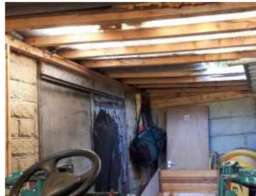
Photograph 8: B4a (internal view)
