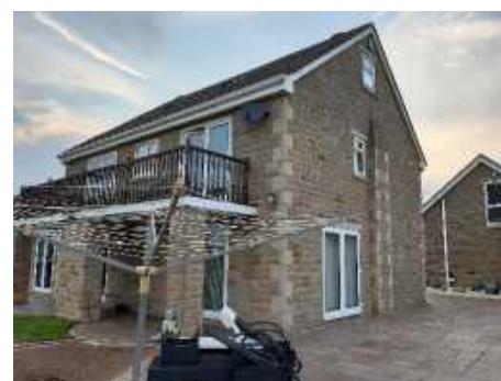
Photograph 12: B7 (showing eastern gable and southern aspect)
