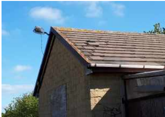
Photograph 7: B4 (southern aspect)
