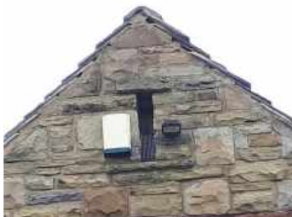
Photograph 9: B6 (gable end roost feature)
