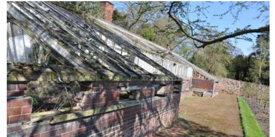
Existing North Range Glass House
