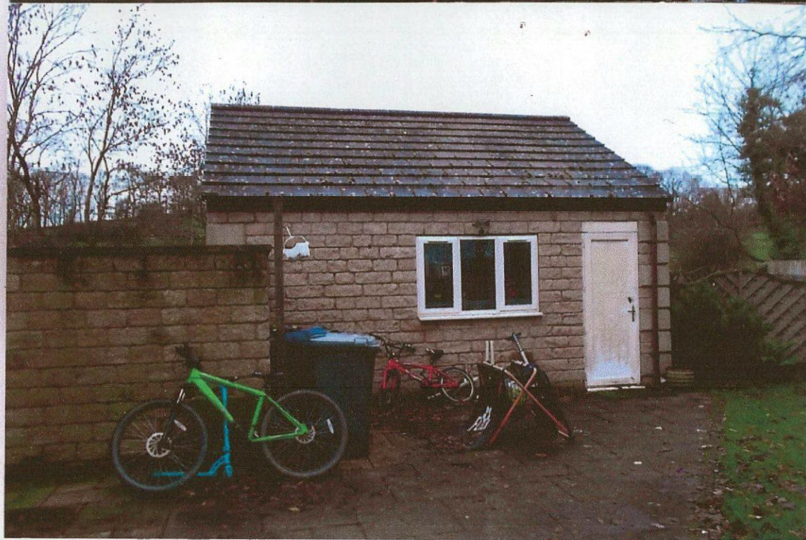
VIEW WITHIN GARDEN CUTLAGE TO REAR
