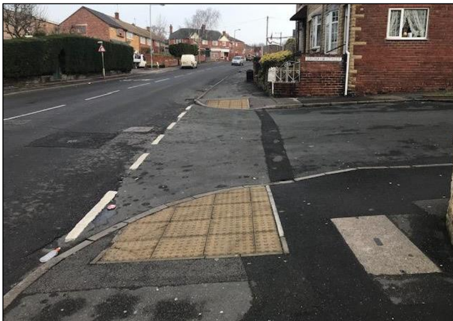
Figure 7. Dropped Kerbs and Tactile Paving North of B6098 Goldthorpe Road
