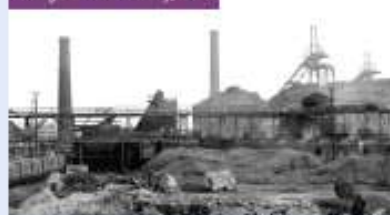
Houghton Main Colliery, 1997
