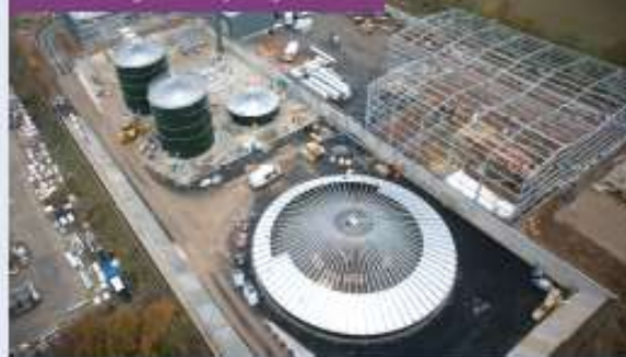
An Anaerobic Digestion facility during construction
