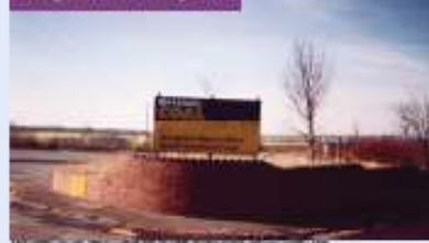
Houghton Main Colliery, 1993
