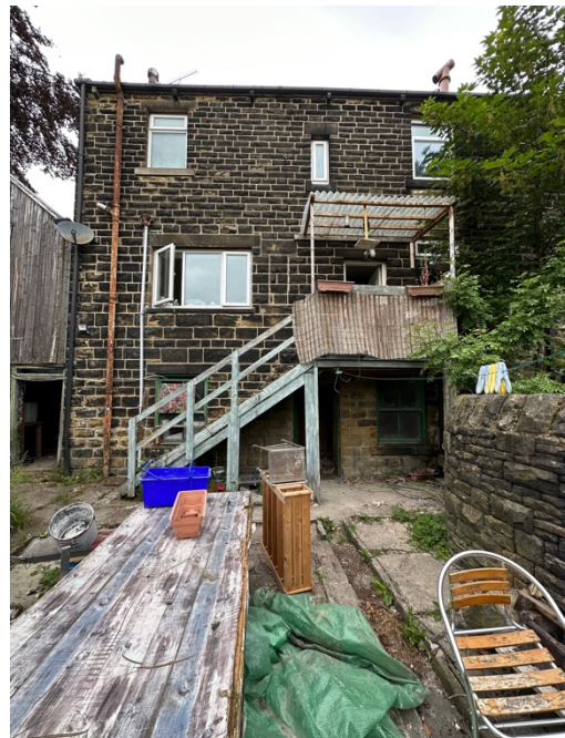
Photo showing the rear with the existing timber stairs and view of the lower ground floor.
