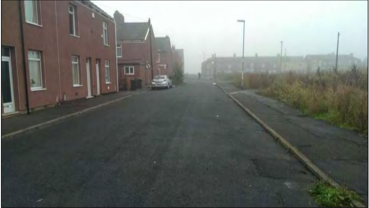
Figure 3.6 – East Street, looking south
