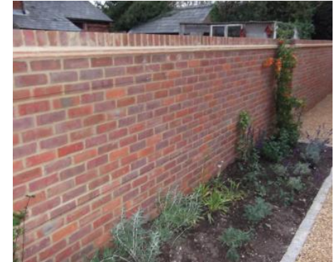
Typical 1.8m high Brick Boundary Wall
