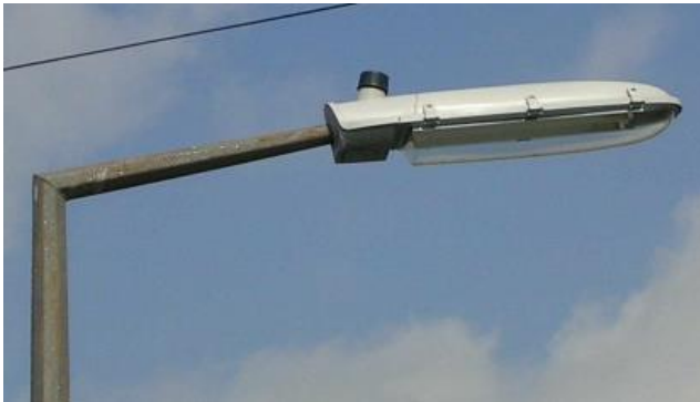
Typical example of Street Lighting
