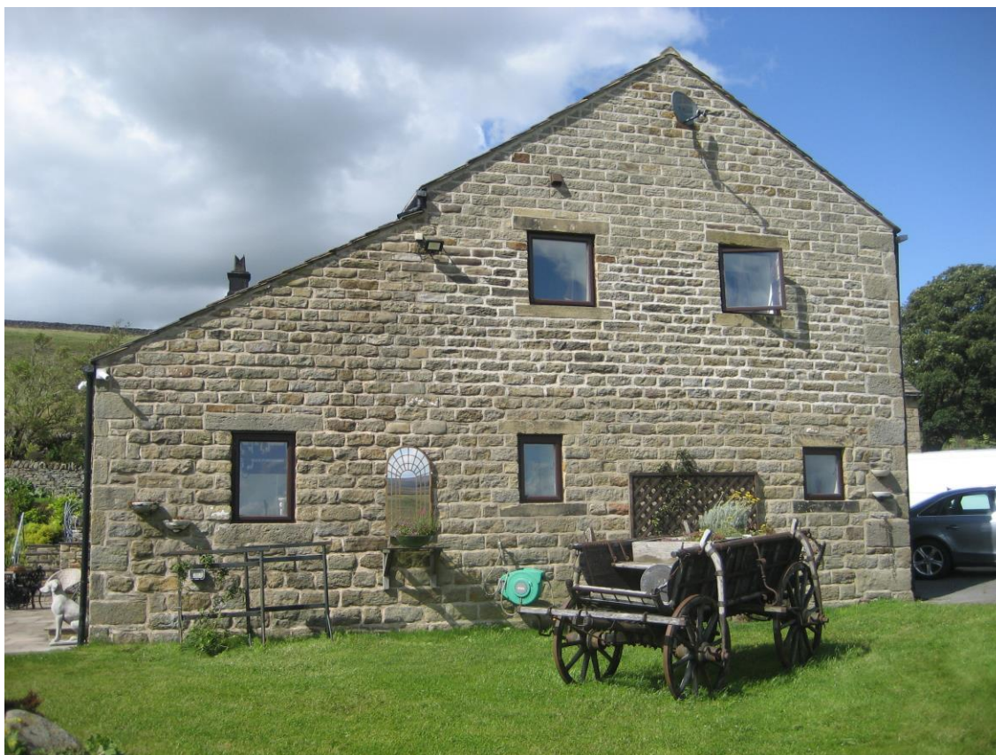
Photo showing south elevation of the previously converted linked barn.
