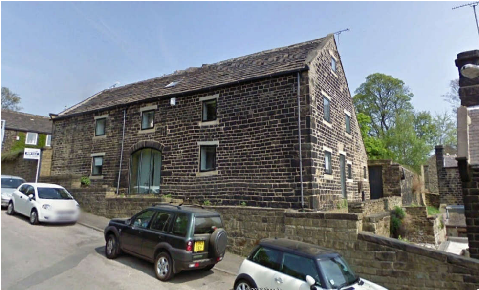
Fig 07. Redminster Barn – West Elevation to Towngate
