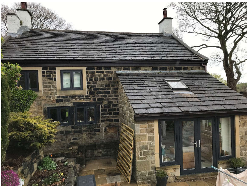
Fig 08. Existing rear lean-to extension to be taken down.
