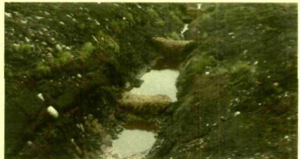
Surface water treatment measures for silt removal
