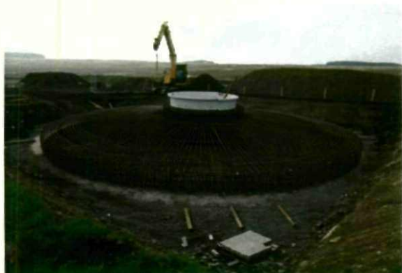
Turbine base construction.
