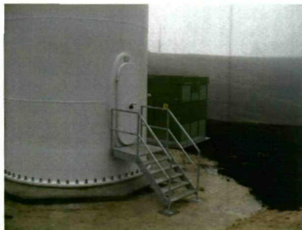
Access to the turbines for maintenance
