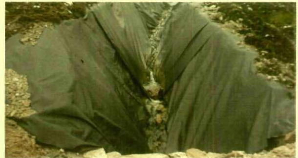
Example of drainage of an existing watercourse
