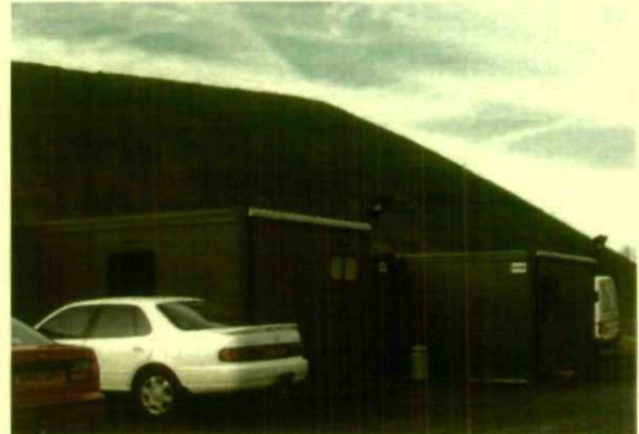
An example site office
