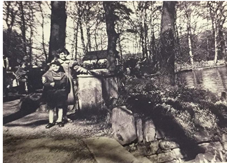
Site 1946 showing boat house
