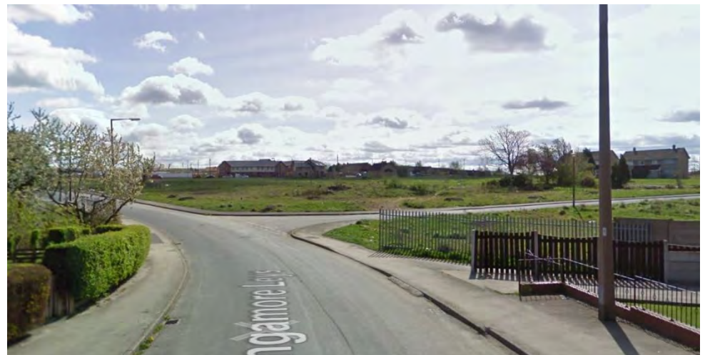
Photo 6. Site entrance – Lingamore Leys
