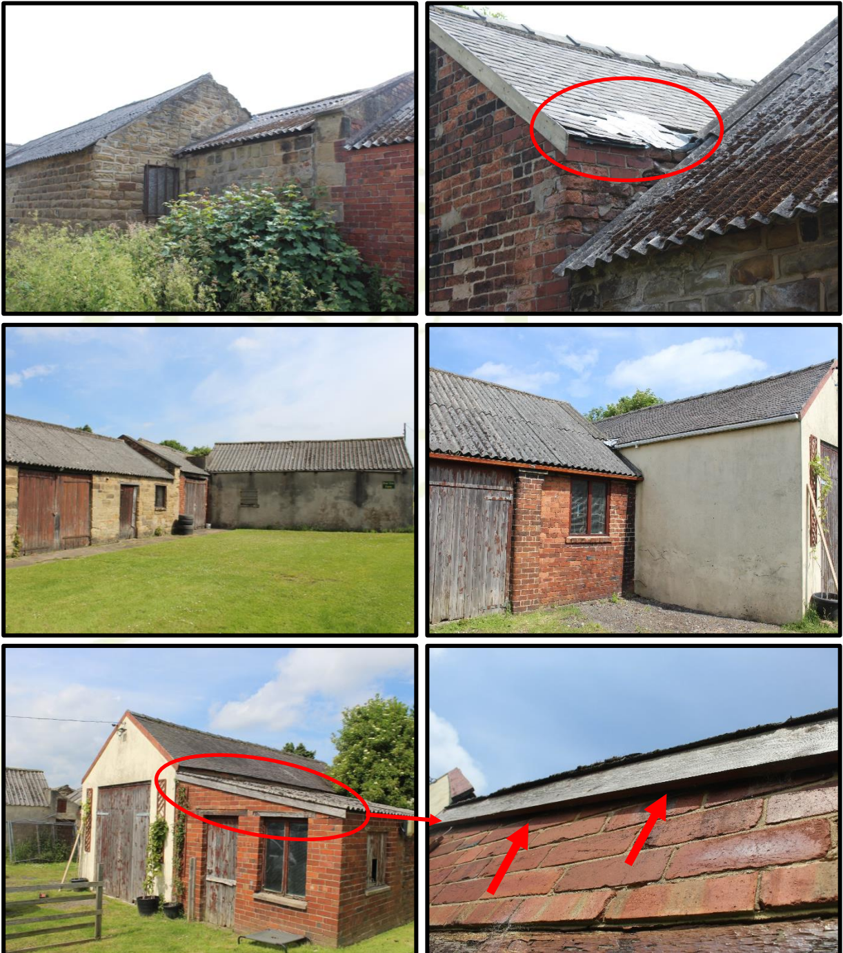
Figure 4: Building Complex (B3) with Potential Roost Features Highlighted
