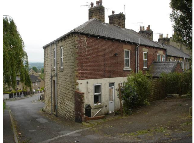
Fig 03. Typical housing adjacent to the site
