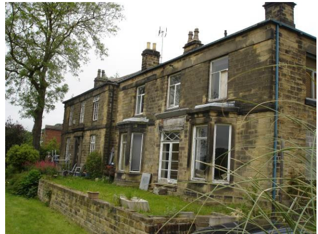
Fig 05. Victorian extension to be removed
