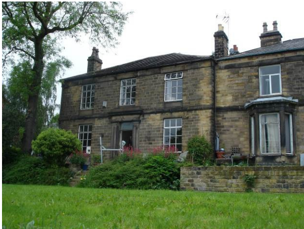
Fig 04. Original Georgian house (left)
