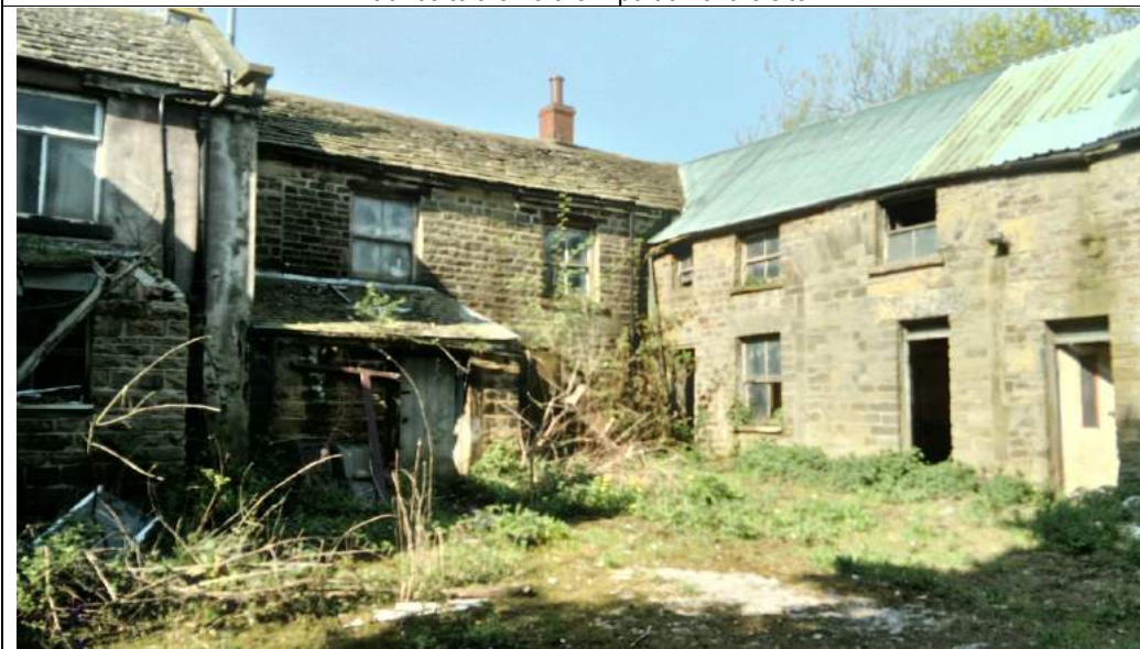
Northern portion of the site
