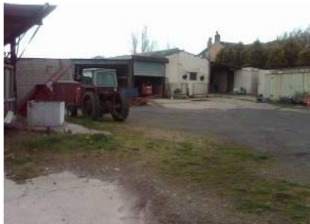
Fig 3.3 – Existing appearance of various buildings.
