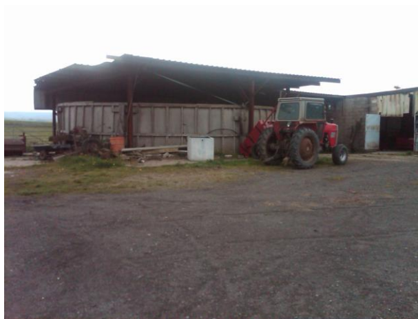
Fig 3.4 – Existing appearance of various buildings.
