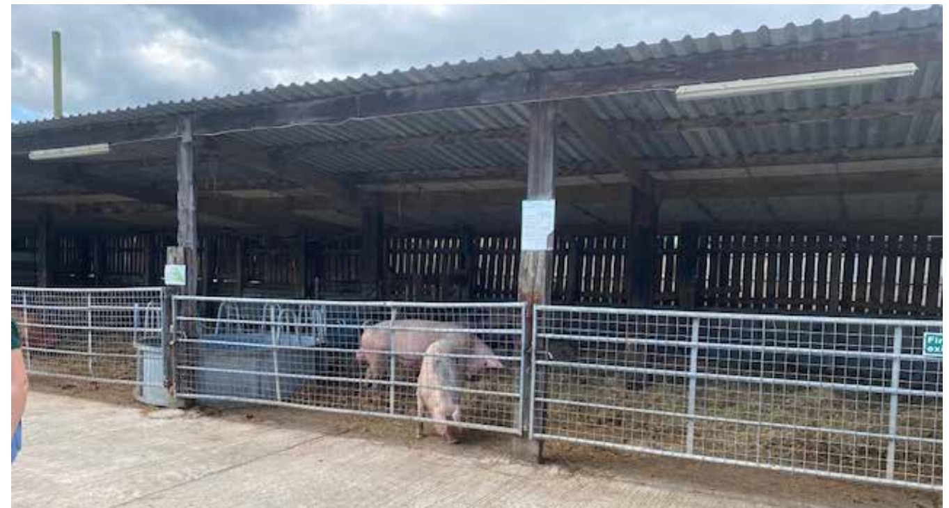
Photograph of East Elevation of existing Livestock Shed from east
