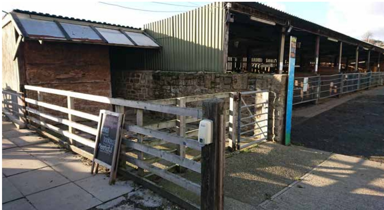
Photograph of East and South Elevation of existing Livestock Shed from south east
