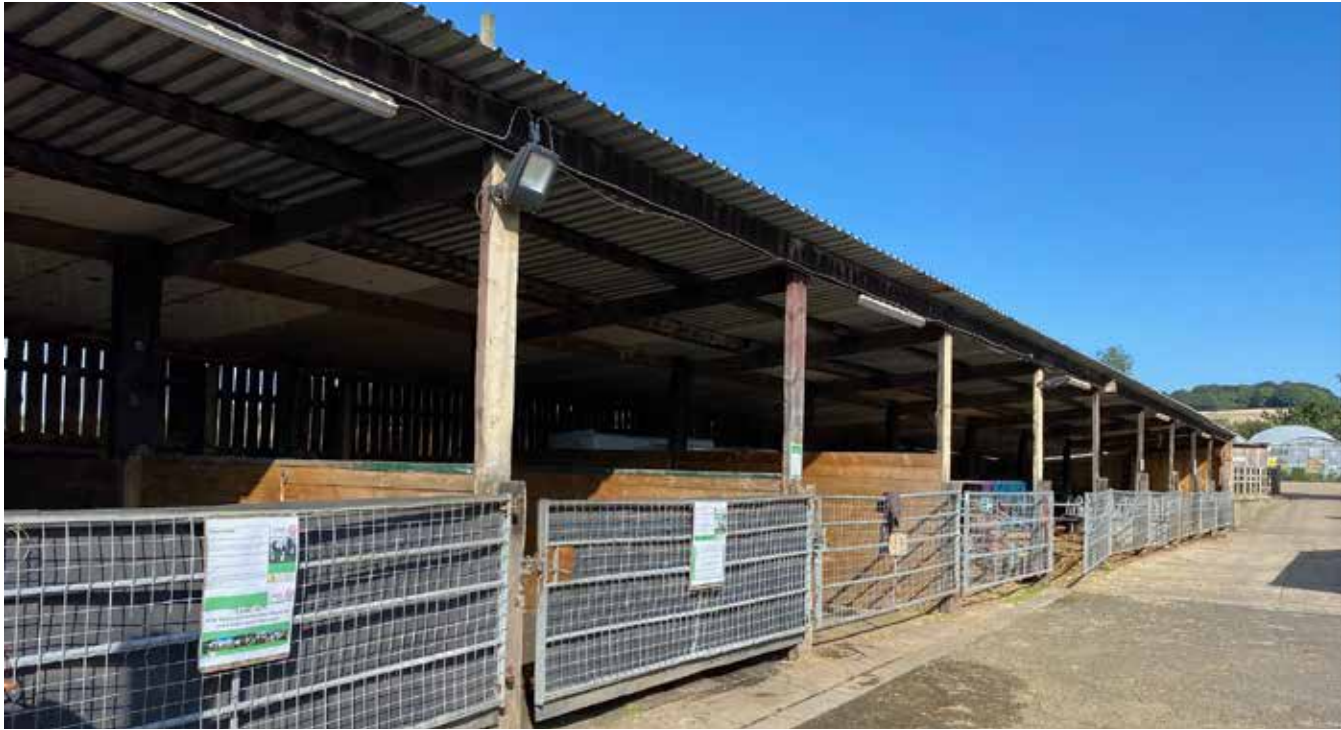
Photograph of existing Livestock Shed at Wigfield Farm campus, Barnsley
