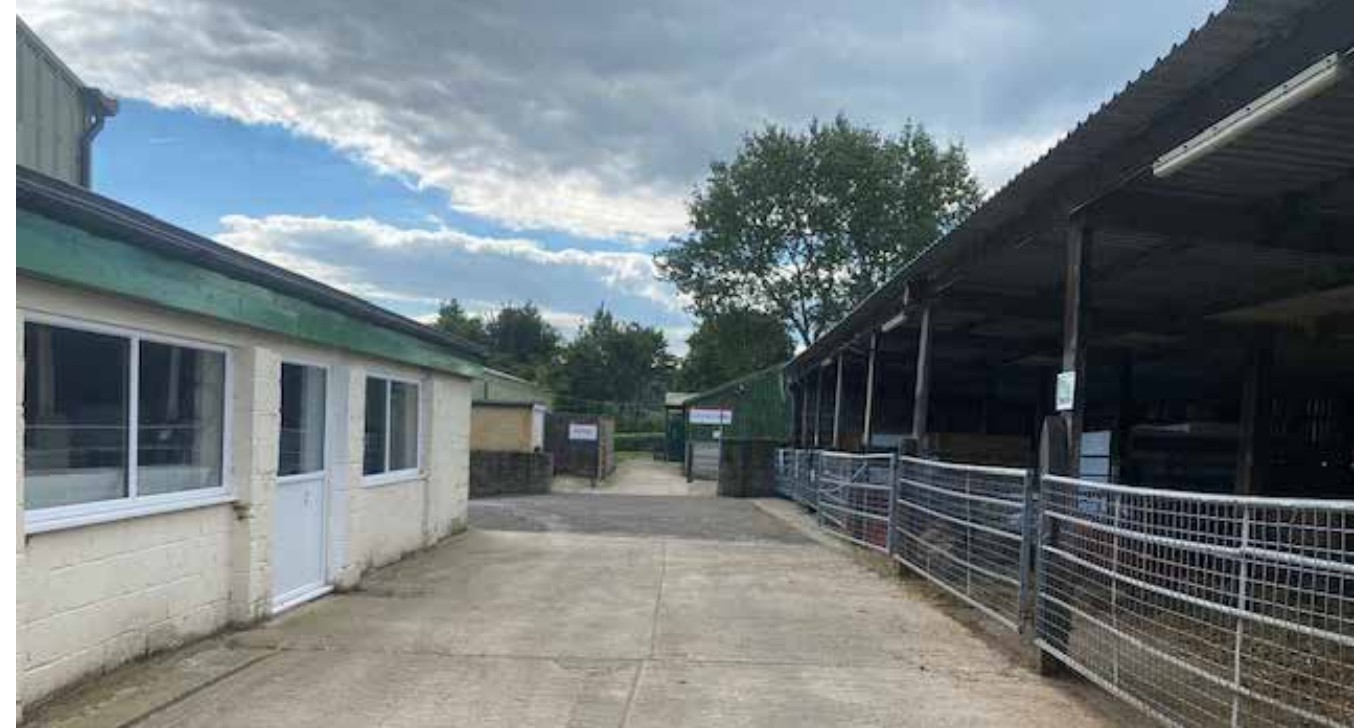
Photograph of East Elevation of existing Livestock Shed from north
