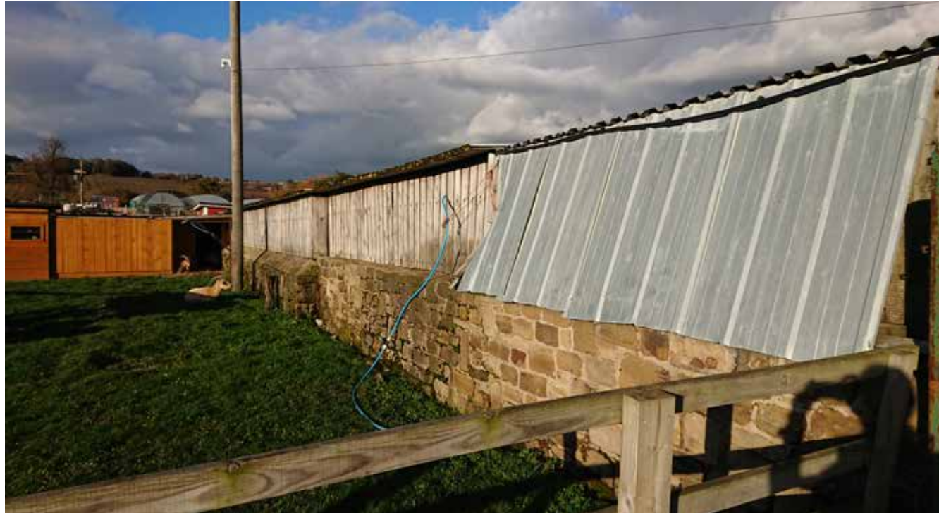
Photograph of West Elevation of existing Livestock Shed from south west
