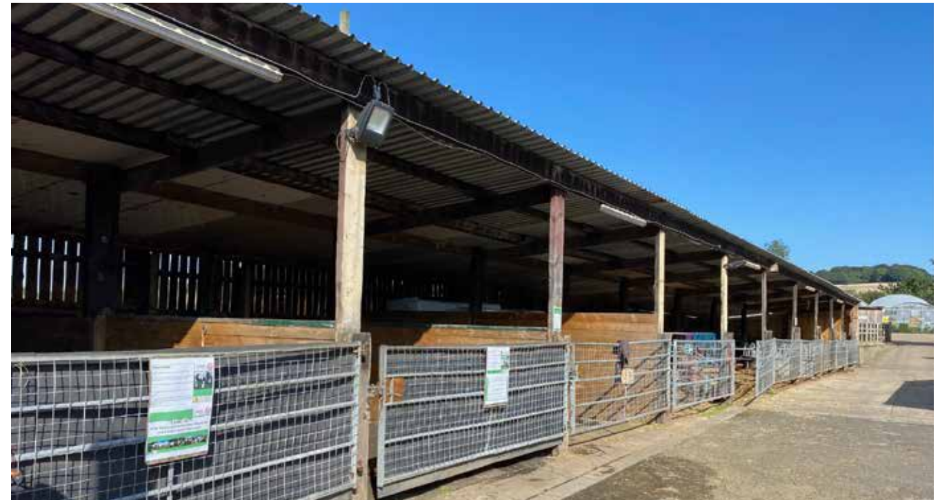
Photograph of existing Livestock Shed at Wigfield Farm campus, Barnsley
