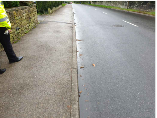
11 - Scarring and fretting on footway. Kerbs damaged and misaligned.
