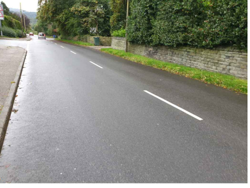
13 - Verge in tact with no damage
