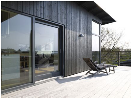
Black Vertical Cladding with Aluminium Doors
