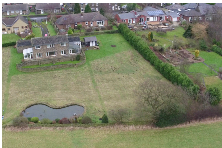
Aerial View of Site from South
