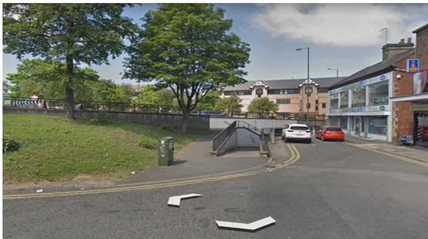
Photograph 2 – Doncaster Road Underpass Entrance
