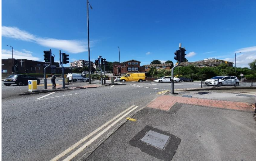
Photograph 2 – Pedestrian Crossing Facility
