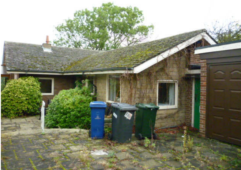
Photo 1: 6 Cliffe Hill, viewed from front
