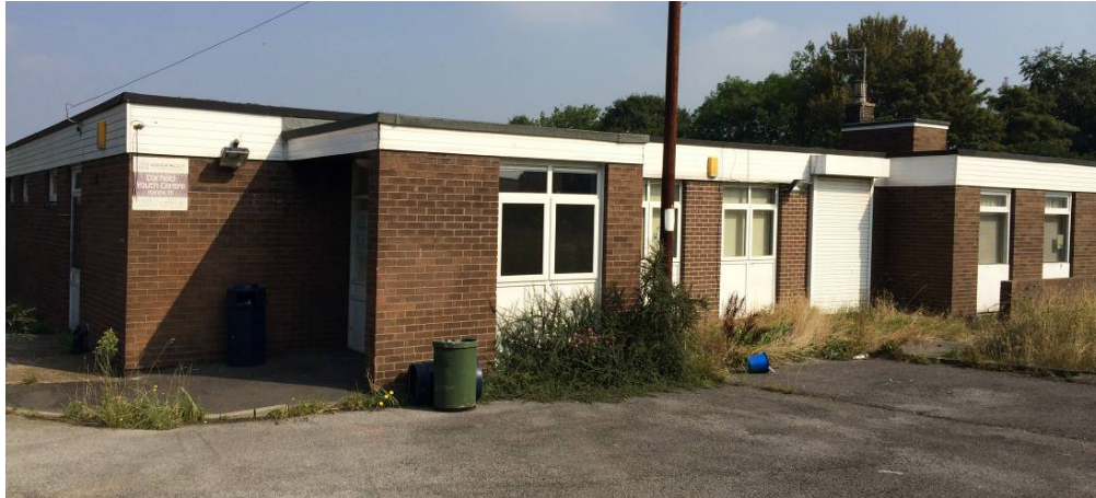
Figure 2 General view of the property
