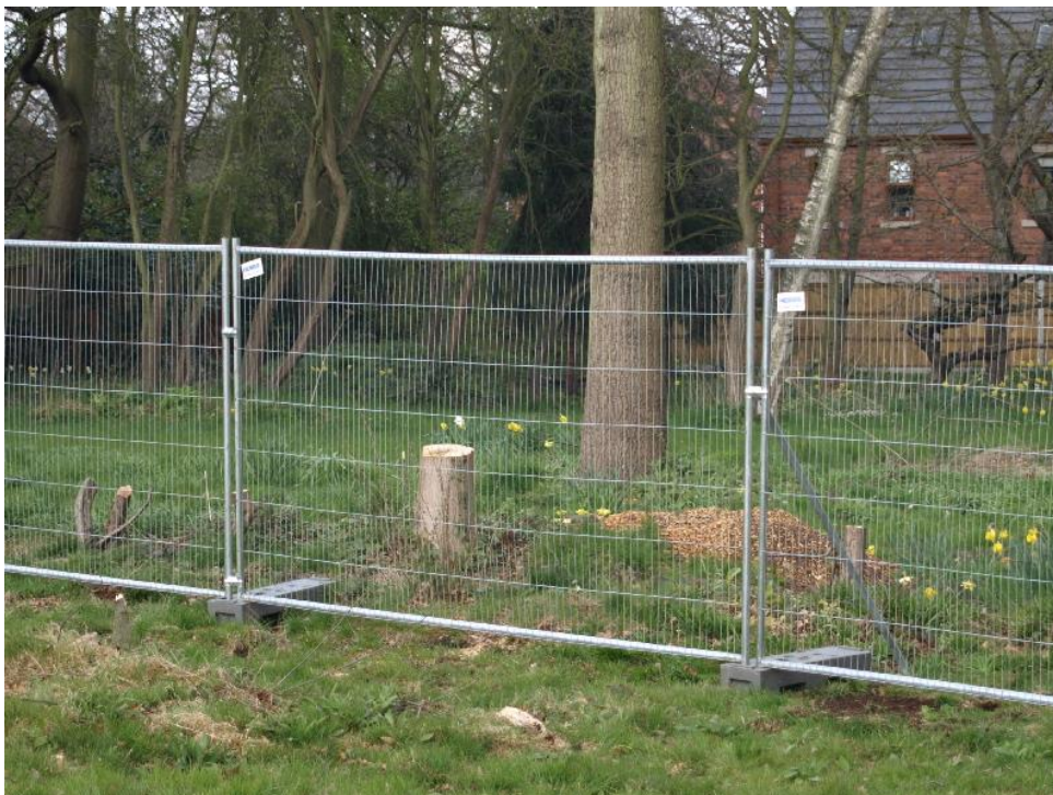
Photograph 12; tree protection fencing.
