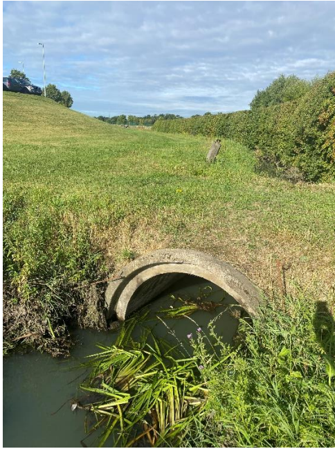
Figure 22. TRIB_004 upstream inlet- 1.35m diameter culvert
