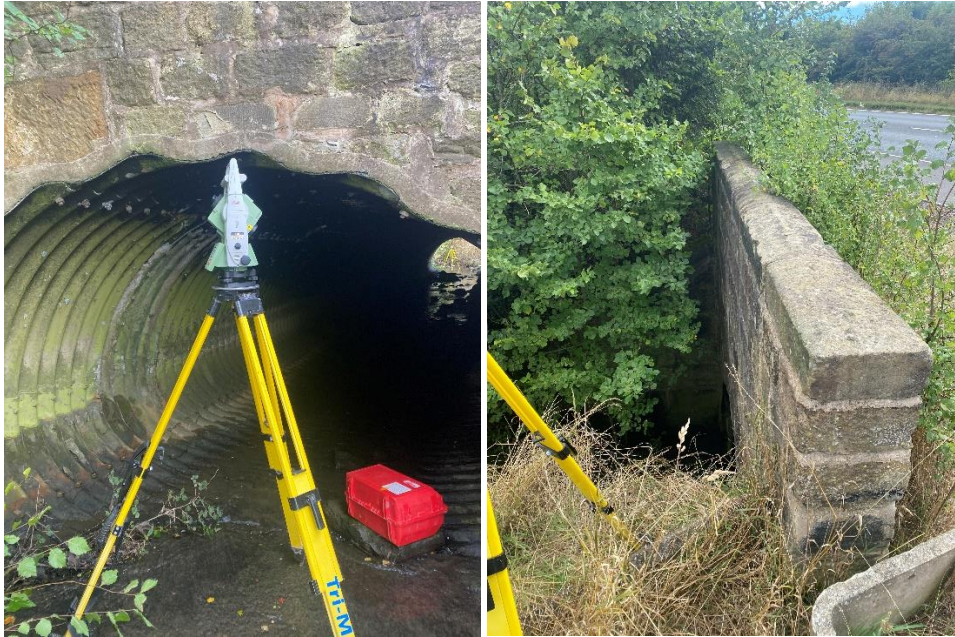
Figure 20. CARR_007 upstream inlet - A635 Culvert
