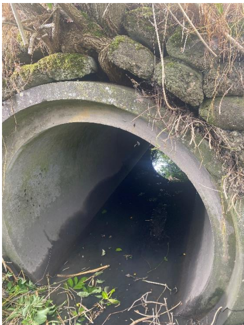
Figure 24. TRIB_011 upstream inlet - 1.5m diameter culvert
