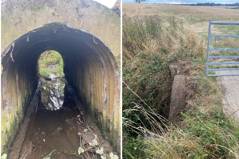
Figure 19. CARR_002 upstream inlet - Farm Access Culvert
