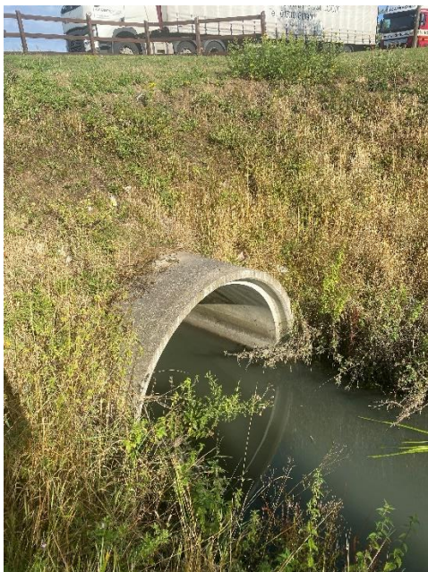
Figure 21. TRIB_002 upstream inlet - 1.9m diameter culvert
