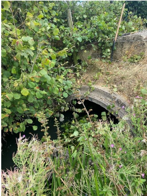
Figure 23. TRIB_007 downstream outlet - 1.75m diameter culvert
