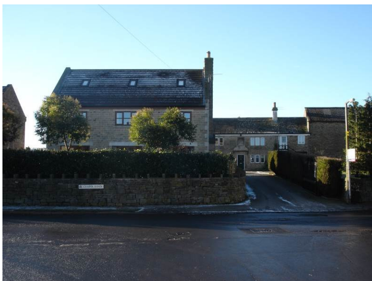
08. Existing dwelling to south east of site
