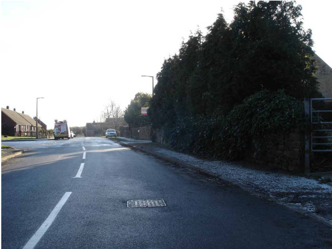
03. View of site frontage to Chapel Road looking south east.
