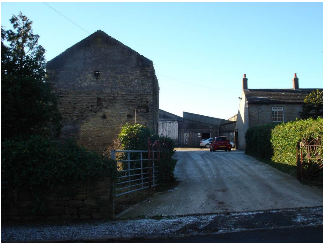
02. View of access to Ivy House Farm looking south west.
