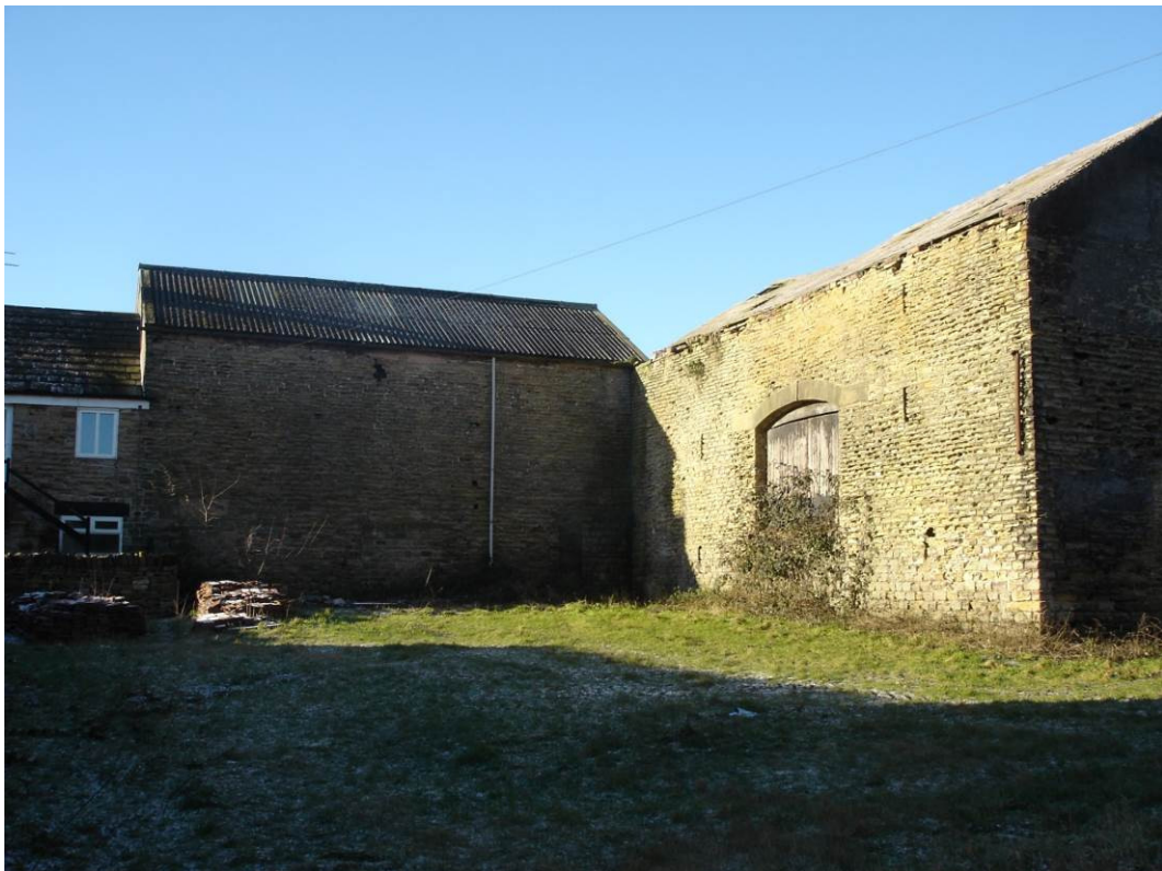
06. View of existing barns to rear looking west.
