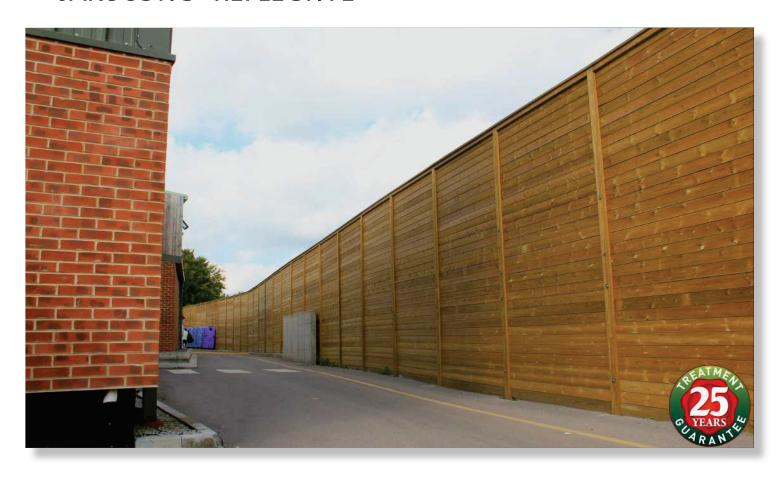
The Jakoustic® Reflective barrier is particularly effective in reflecting noise away from its face by employing heavy section planed timber boards with deep interlocking 'v' tongue and groove joints, coupled to tuning fork posts that clamp the boards together to eliminate gaps that sound could easily travel through.
