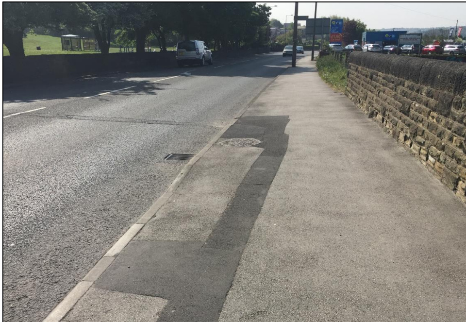
Image 2.2 Wakefield Road – View looking South
