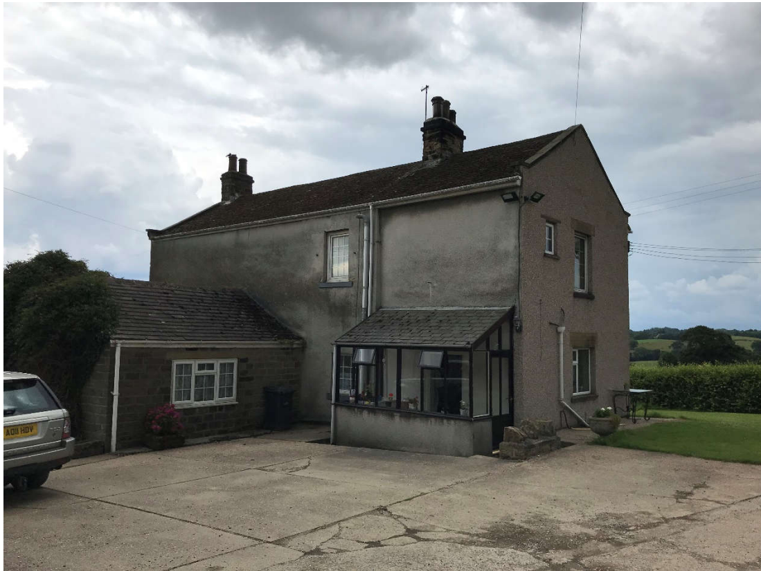
Fig 01. Farmhouse North Elevation with render finish.
