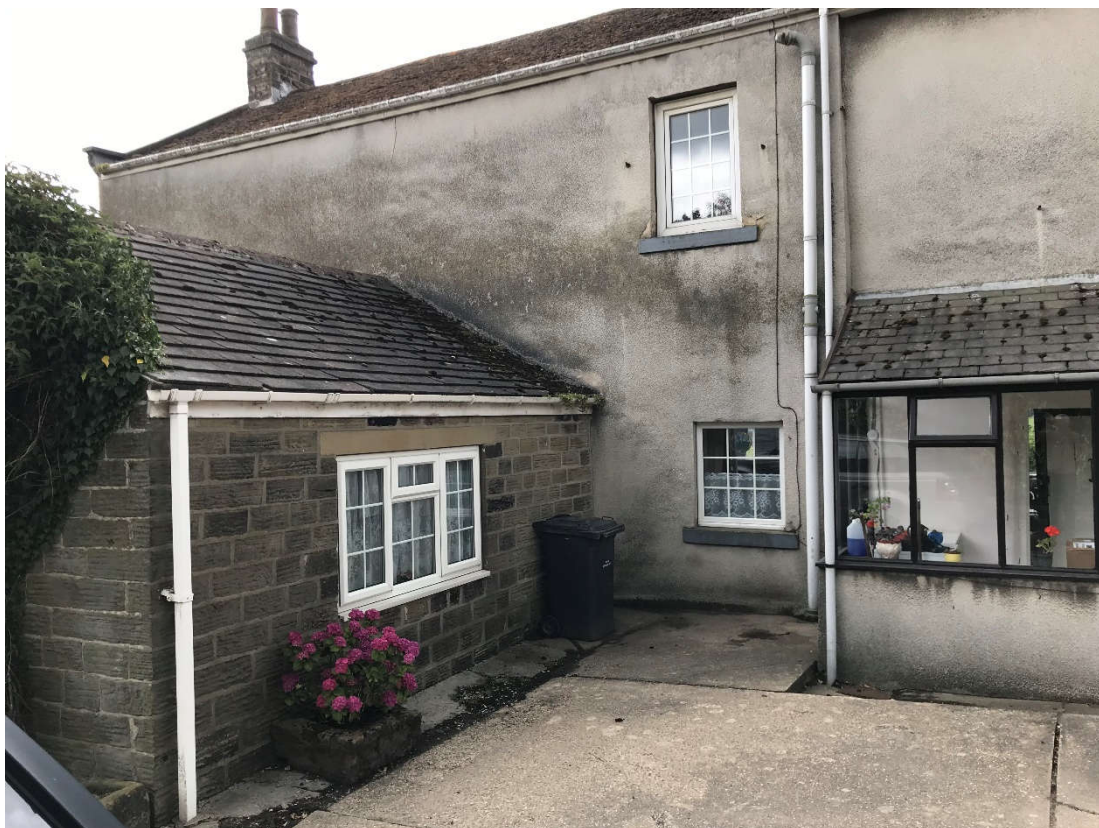
Fig 02. Close view of Farmhouse north elevation and single storey wing to left.
