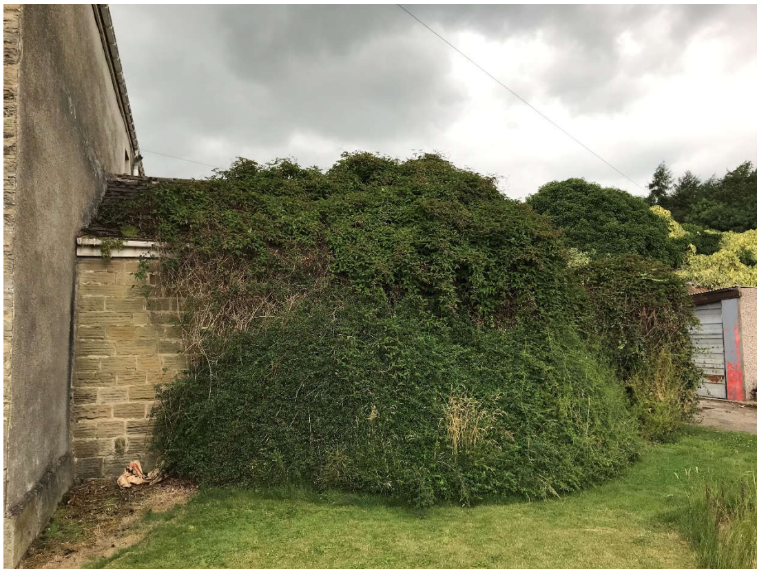
Fig 06. East elevation of single storey wing to north of farmhouse.
