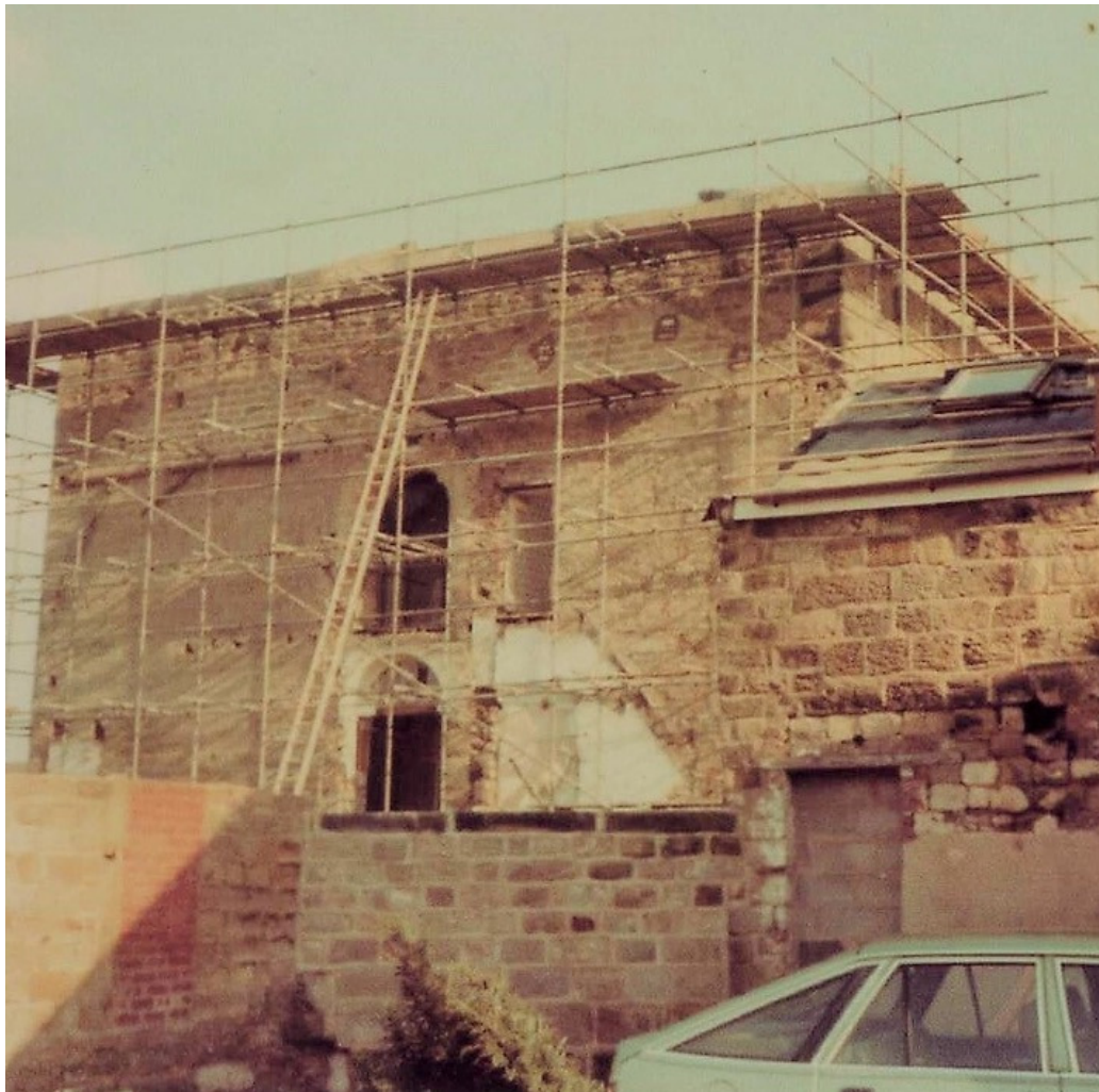
fig. 5 - previous two storey rear extension demolished – arched Georgian doorways and windows were subsequently blocked up.
