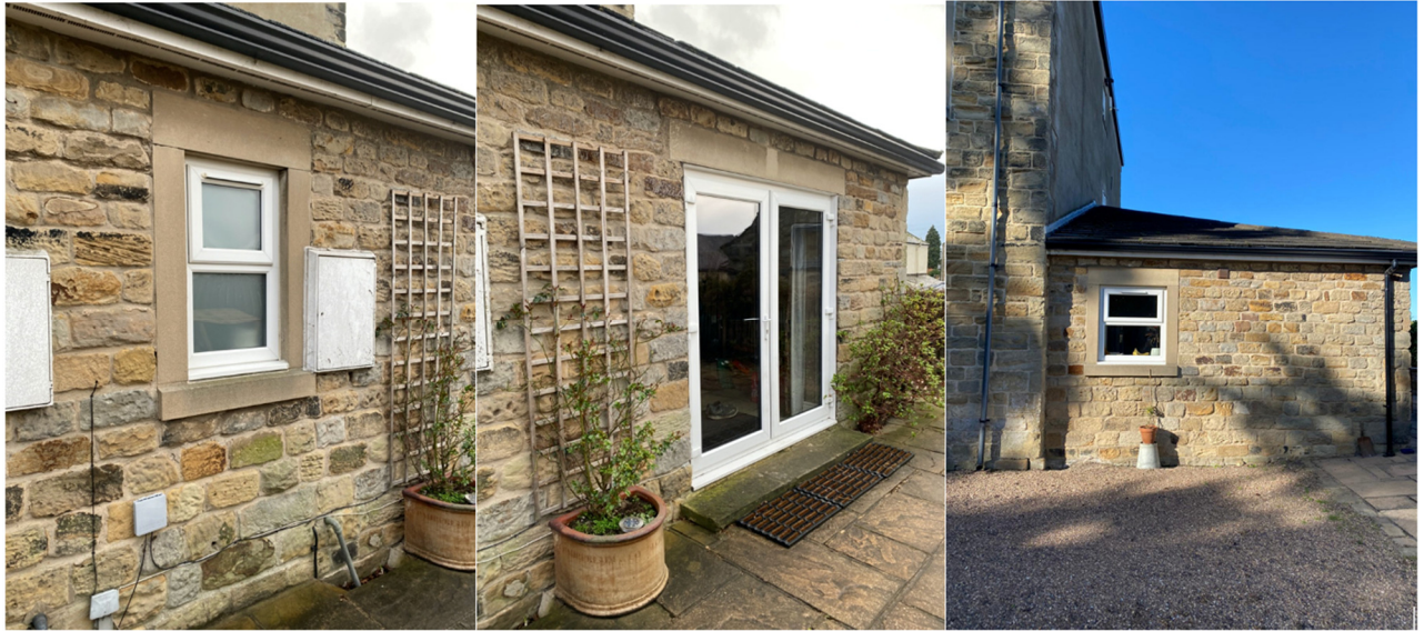
fig. 6 - The 1980s single-storey extension with small white UPVC windows and doors.
