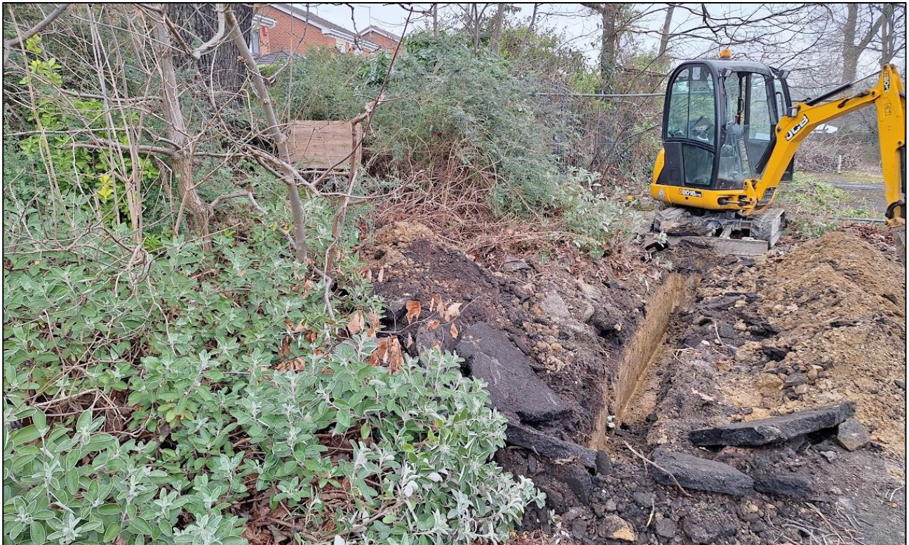
Figure 4: Investigatory Trench Inspection
