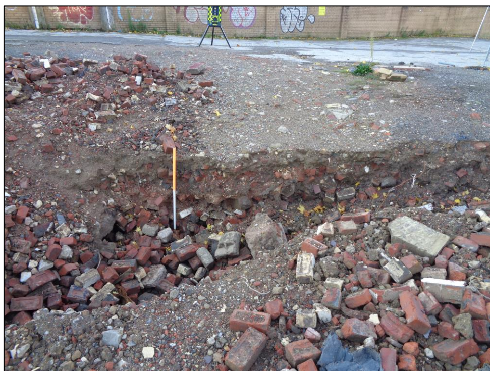
Plate 5: View S showing section of trench backfilled with demolition rubble
