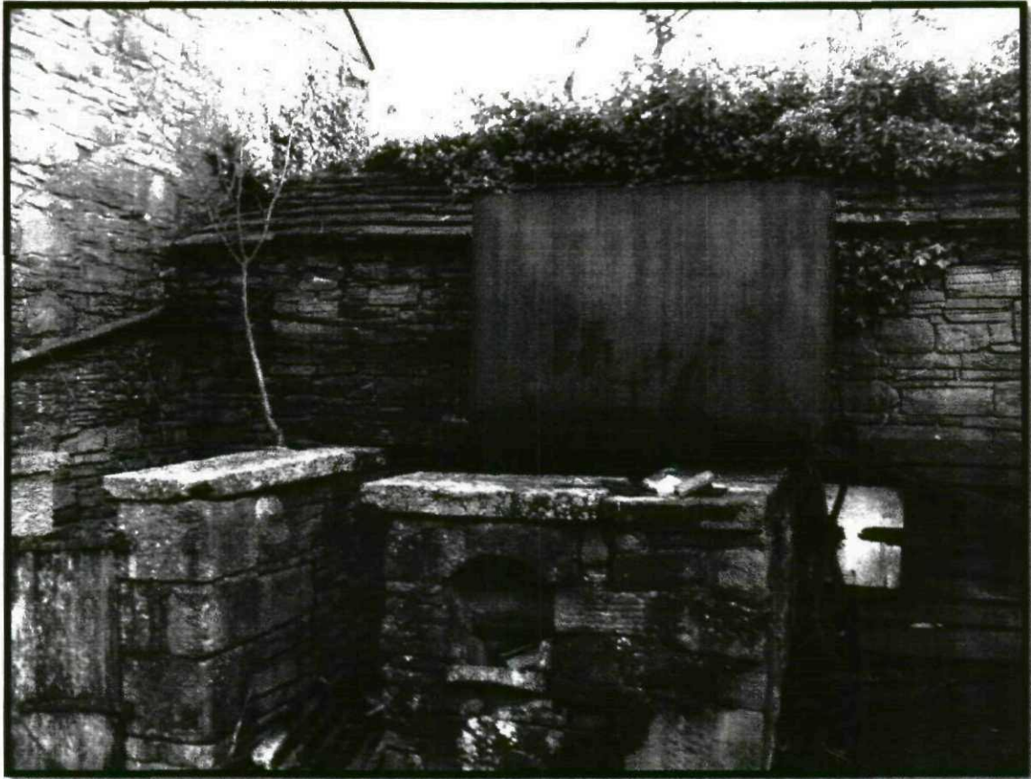
Photograph 55 – View of structure adjacent to the Tractor Shed
