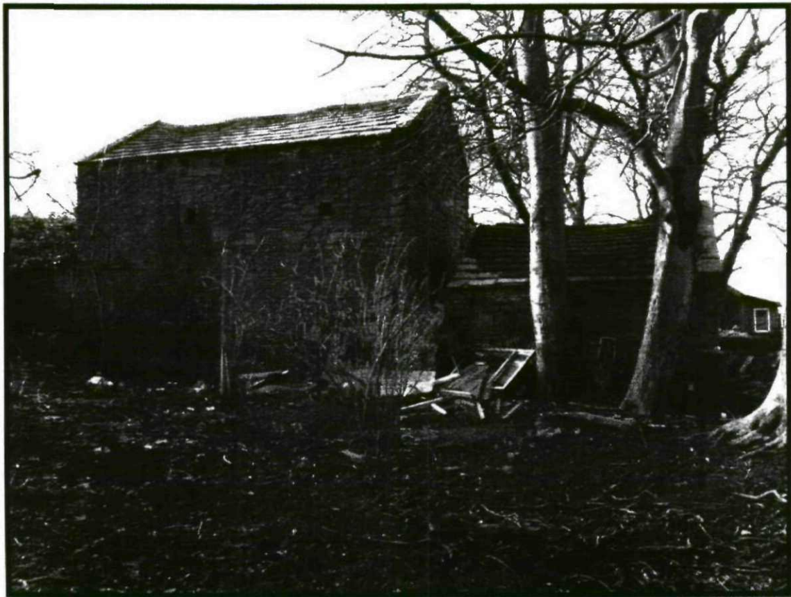
Photograph 50 – View of East Elevation showing trees
