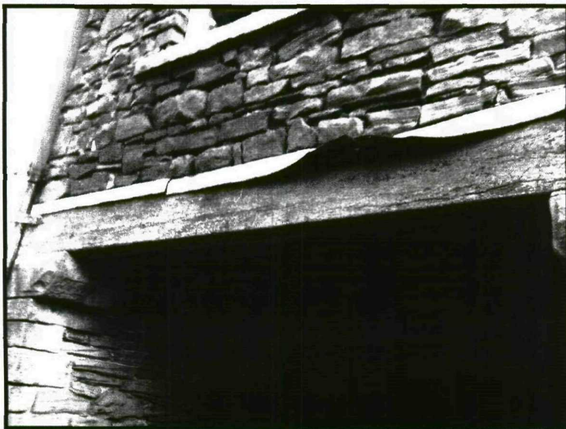
Photograph 54 – View of timber beam tom West Elevation
