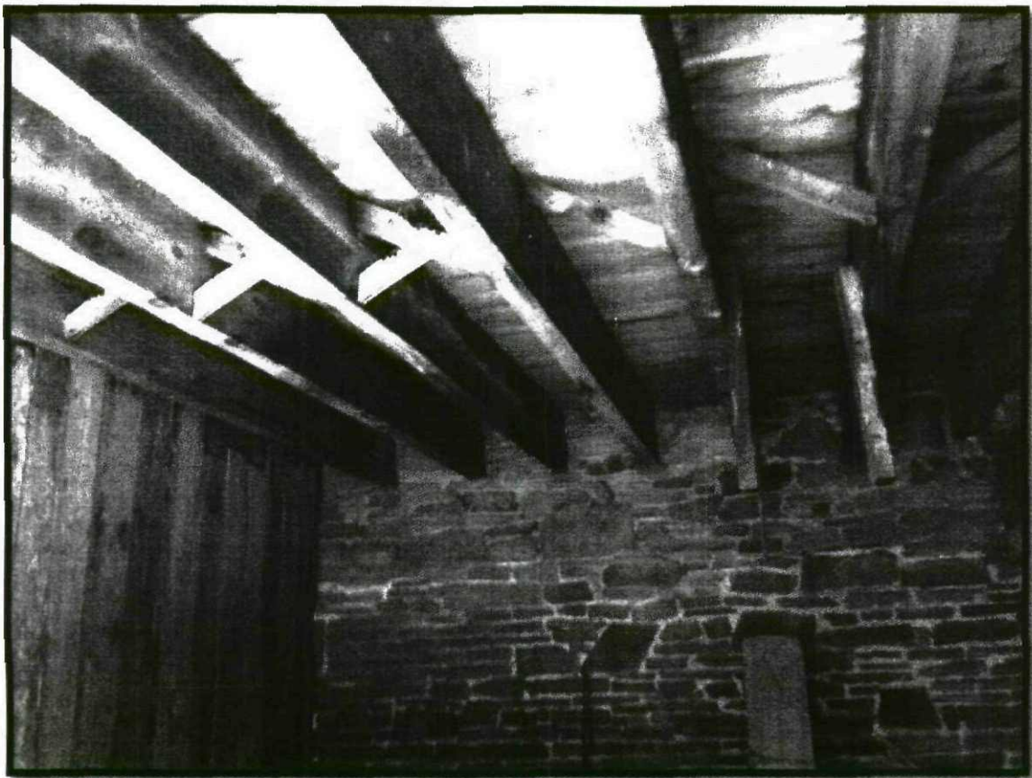
Photograph 60 – View Internal wall construction
