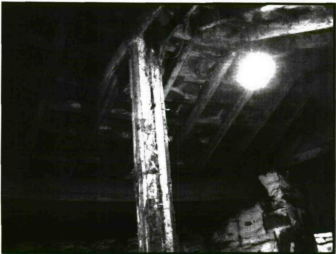
Photograph 68 – View of Annex Roof
