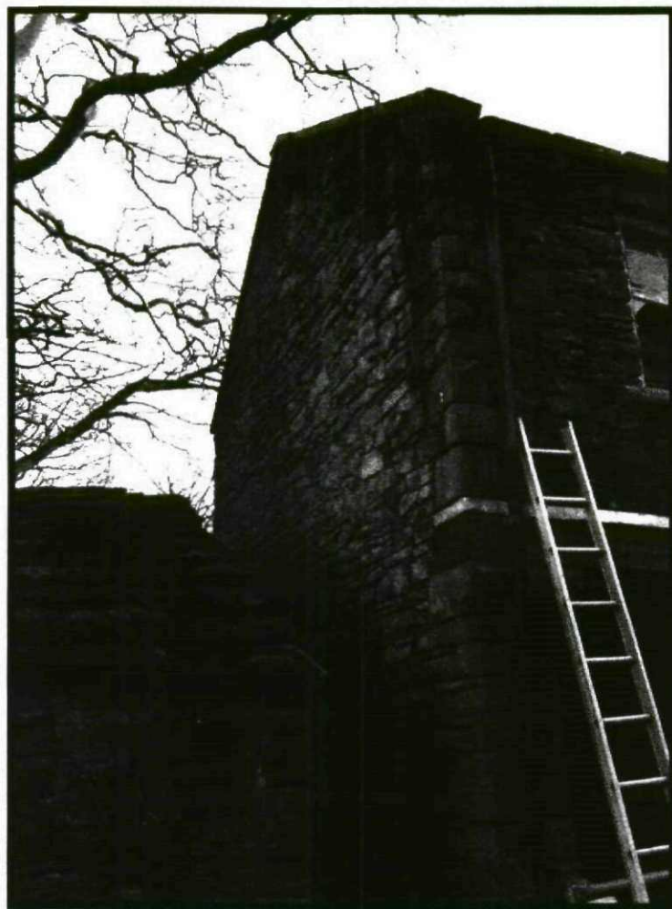
Photograph 57 – View of North Elevation
