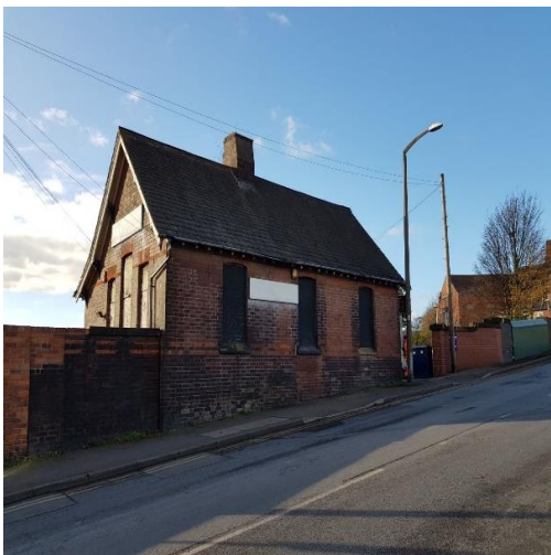
Figure 4: The former ticket office
