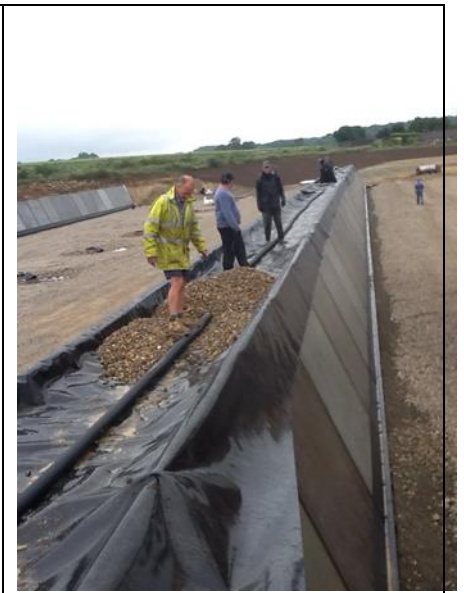
Laying impermeable membrane
