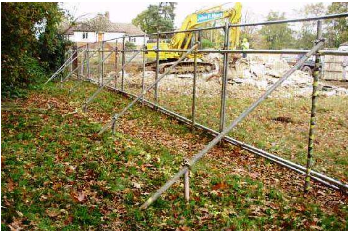
Figure 2: Photo of Fencing to BS 5837: 2012
