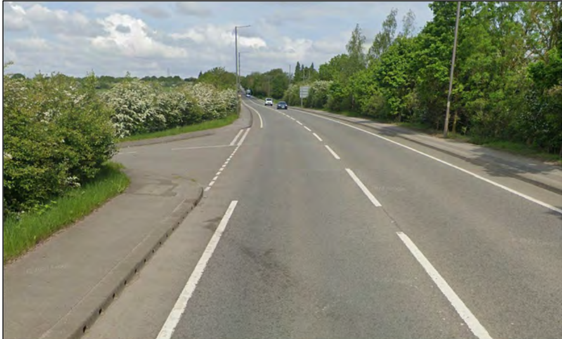
Figure 2.3: Ferry Moor Lane / Engine Lane Junction
