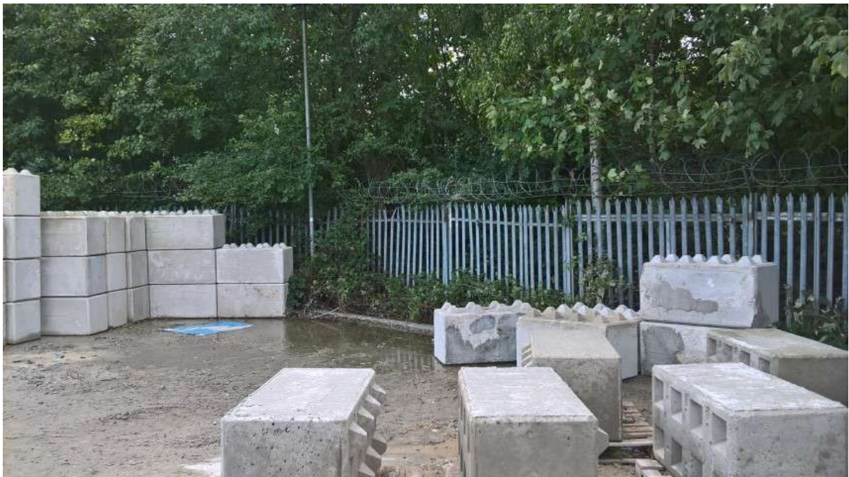
7. South/south-eastern corner of the site.
