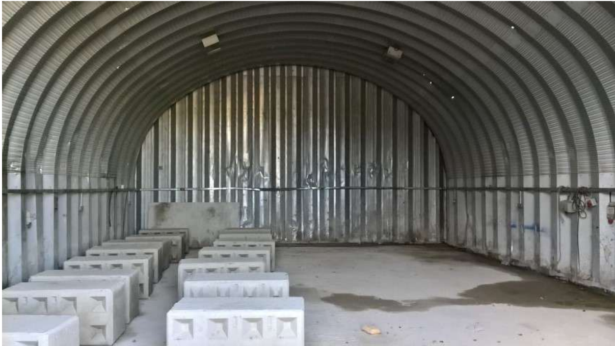
12. View inside the corrugated steel sheet clad building on the site.
