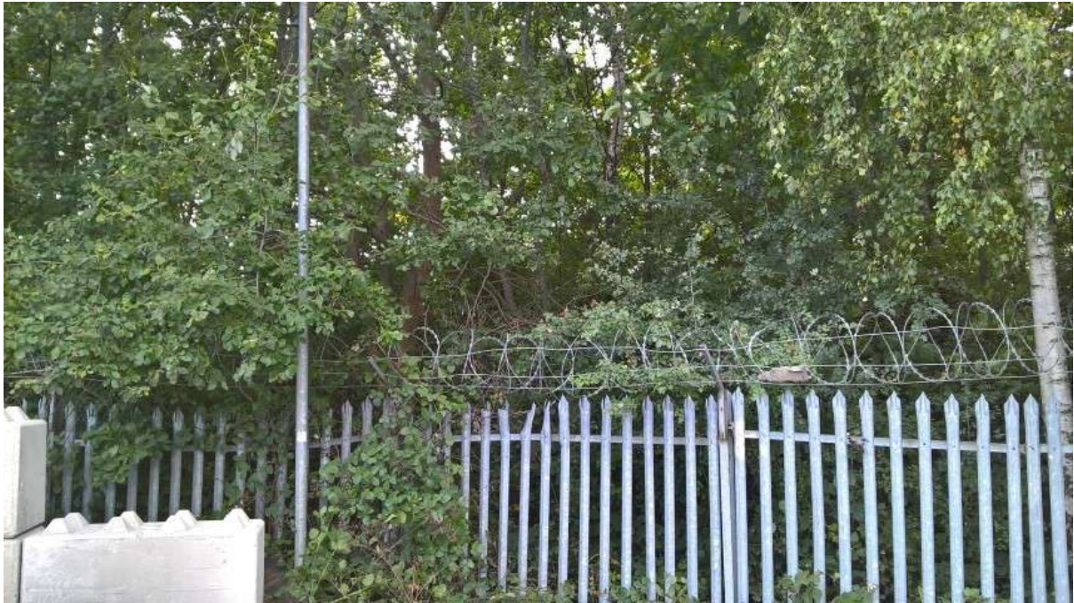
8. Palisade fencing along eastern site boundary. The trees are located on a railway embankment rising to the east from the site boundary. The line is disused and the track removed.
