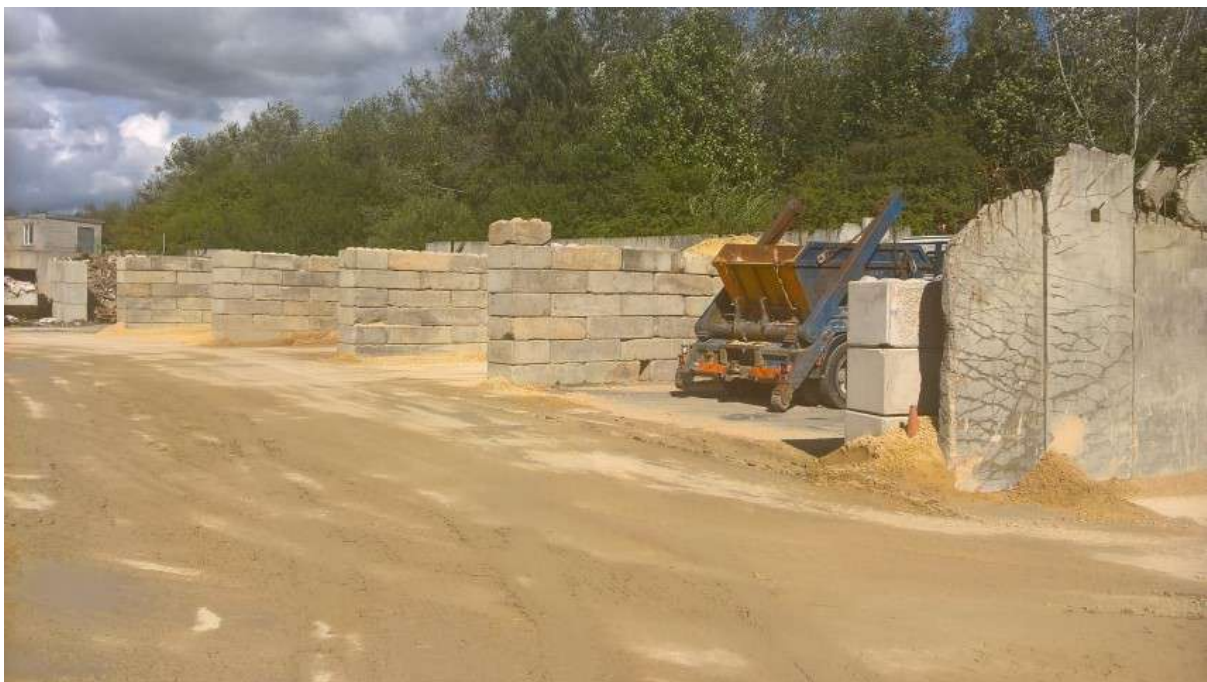
28. Aggregate storage bins along the eastern boundary of the DTS Waste Management site.
