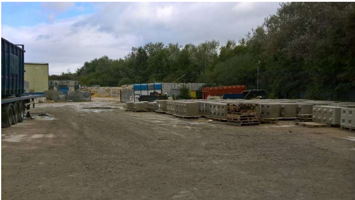
1. View south to north across site, showing concrete block product storage.
