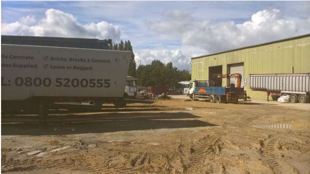
29. View west across DTS Waste Management site, from the aggregate storage bins.
