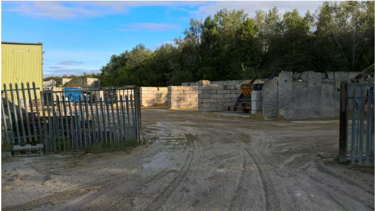
16. Alternative access into the site from the north through the yard area to the north of the site.
