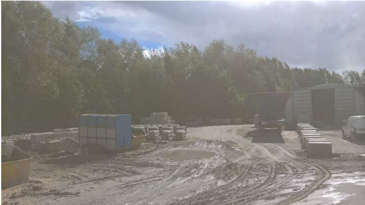
18. General view south/south-east across the site from near the northern boundary.
