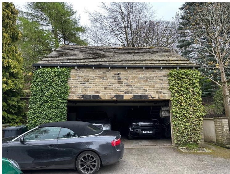
Above Image – Existing Garage
