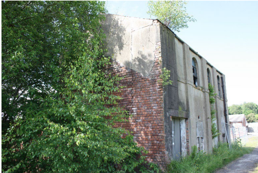
Plate 5: Eastern elevation of principal building, showing crack in brickwork and render
