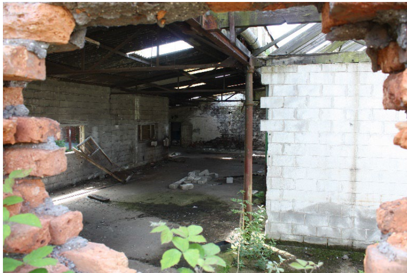
Plate 10: Shot of the workshops showing concrete floor and 20th century blockwork
