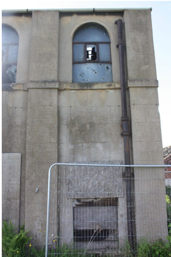
Plate 4: Principal building northern elevation western most bay
