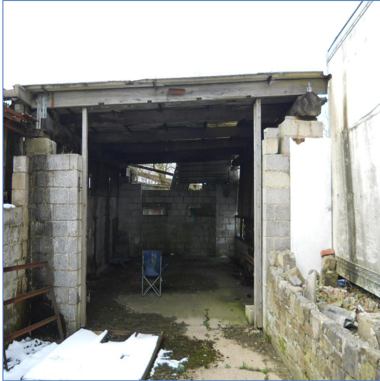
Figure 9: Building 2 (B2) exterior.
