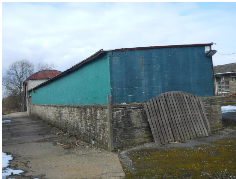
Figure 18: Building 6 (B6) southwest and southeast elevations.
