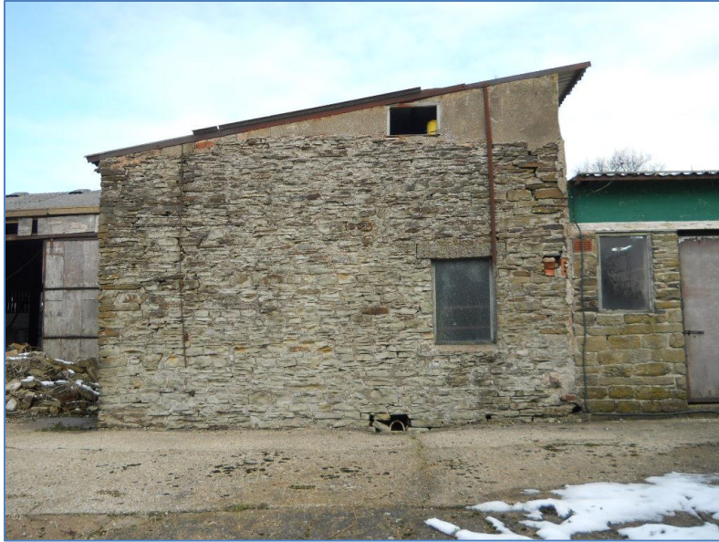
Figure 17: Building 5 (B5) unglazed window on southwest elevation.
