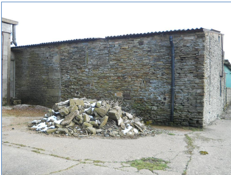
Figure 14: Building 5 (B5) northwest elevation.
