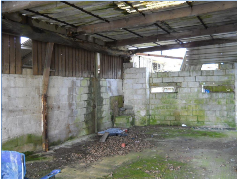
Figure 10: Building 2 (B2) interior.
