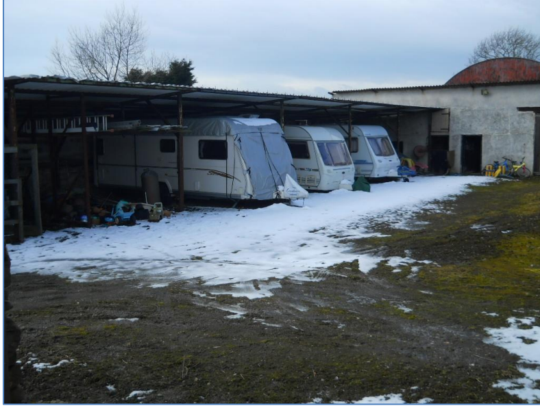
Figure 19: Building 6 (B6) northeast elevation.
