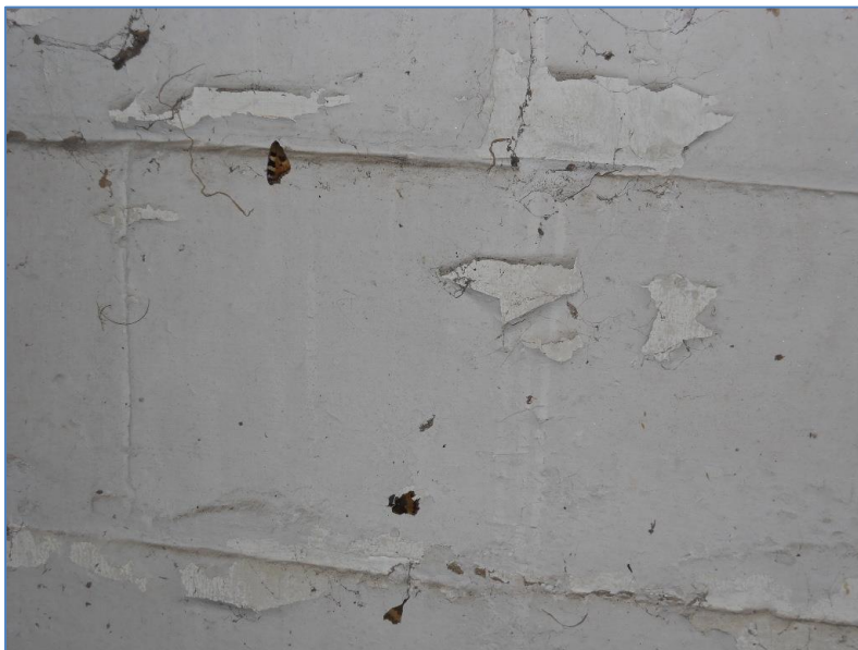
Figure 8: Prey remains stuck in cobwebs below internally boarded window.
