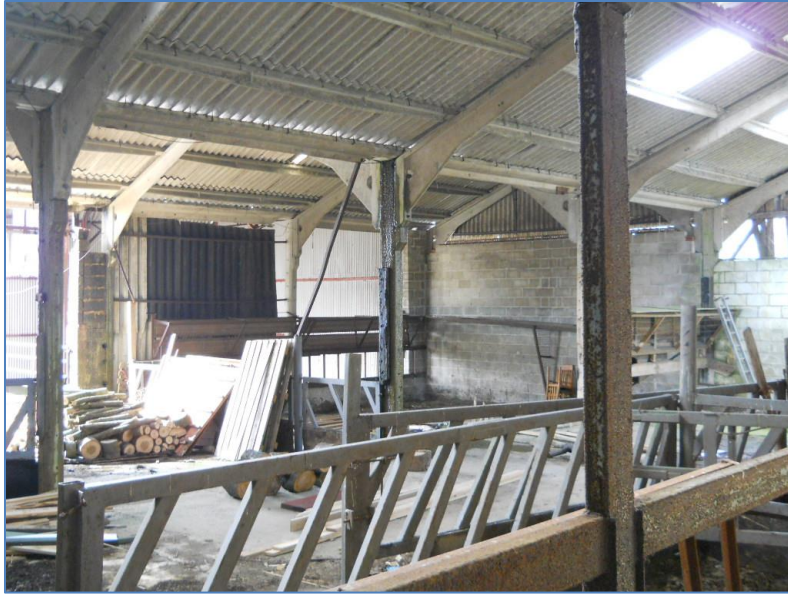
Figure 11: Building 3 (B3) interior.
