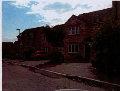
Above: Properties on Cypress Heights access road part of previously completed development.
