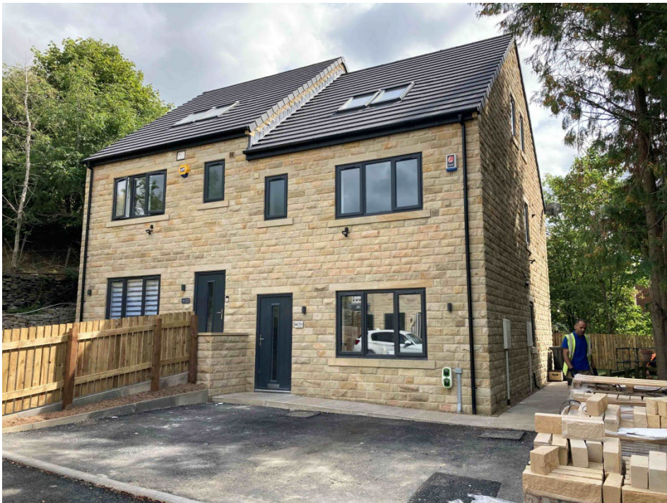
Image 1 - Marley Mini Stonewold Concrete Tiles and Quintanar Sandstone Walls (Previous Houses by Developer Under Construction)
