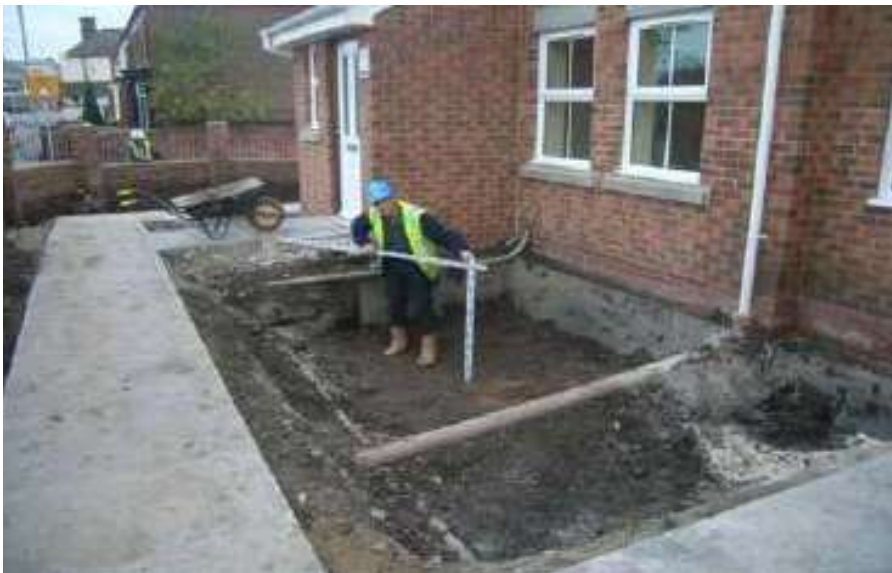
Photograph 4: Depth check of inert cover within areas of front gardens.
