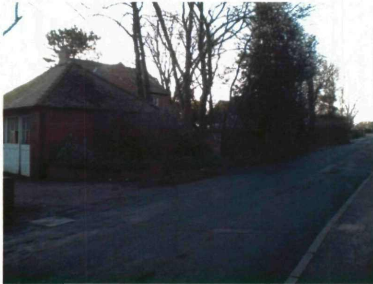
Existing site entrance to be closed
